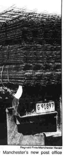
If it rains on the day of the fes- CONCRETE FOUNDATION - Carl Bouley of South mesh for concrete work for Manchester's new post office Windsor, a truck driver for Capitol Steel Co., unloads steel building on Sheldon Road.
